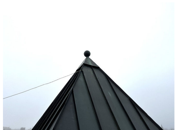
Roof and Pinnacle
