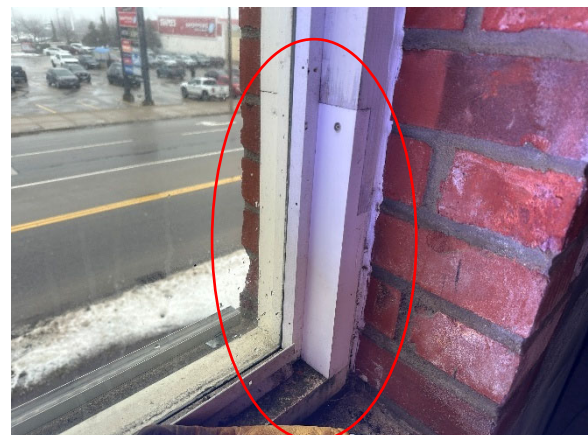
Window Frame Dutchman Repair
