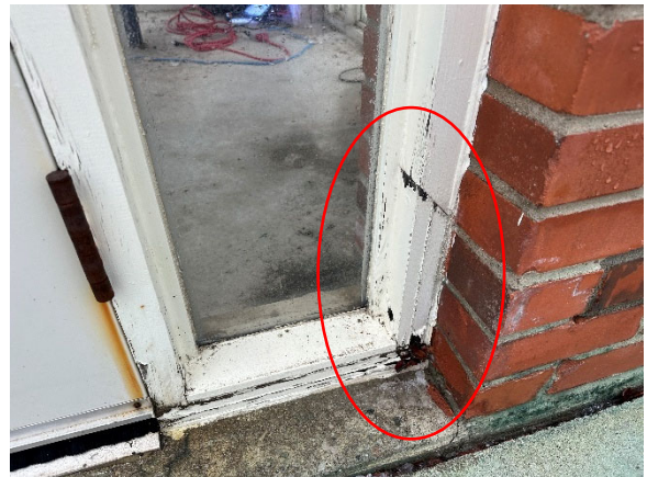
Wood Entrance Screen Deterioration Wood dutchman repair
