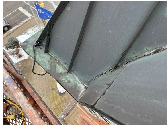
Copper Roofing at Eave and Barrel
