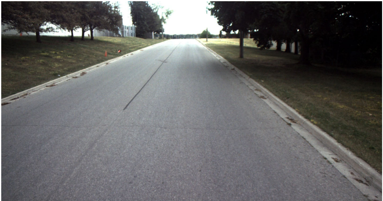
Pavement Condition Good – PCI 75 – 85
