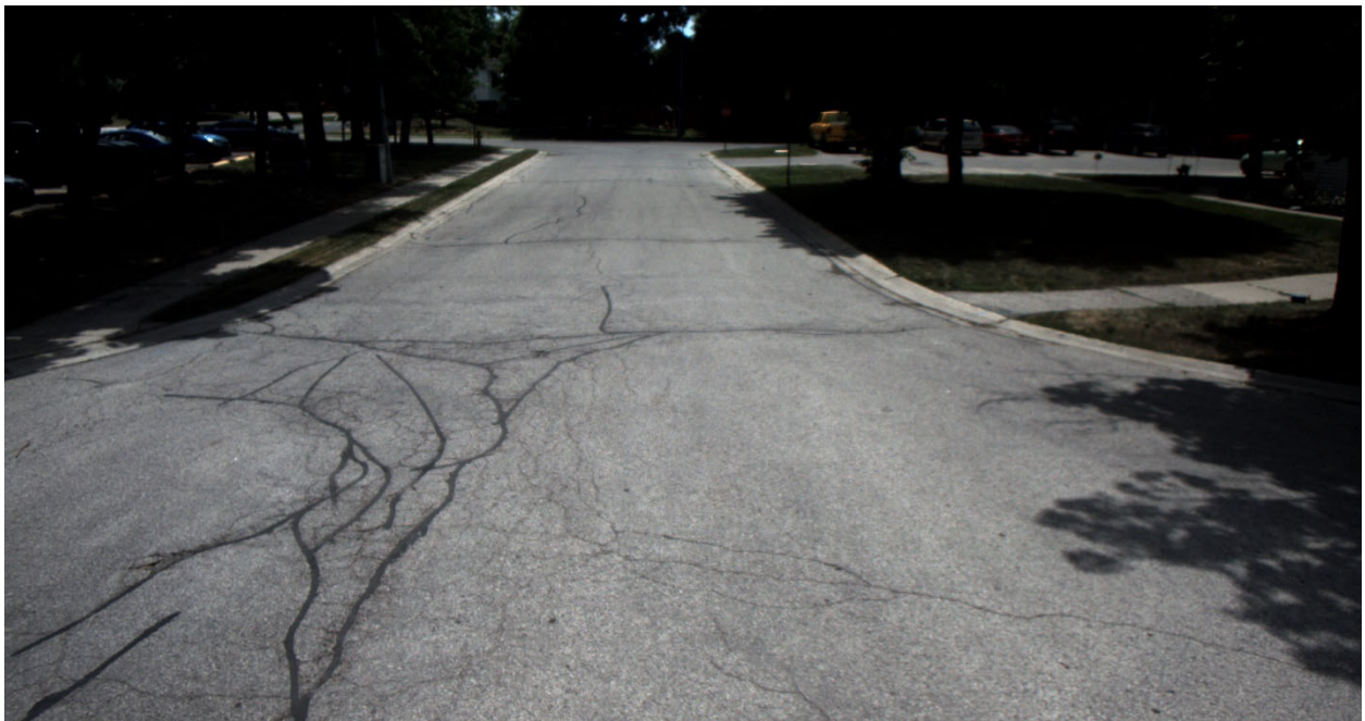
Pavement Condition Poor – PCI 40 – 57
