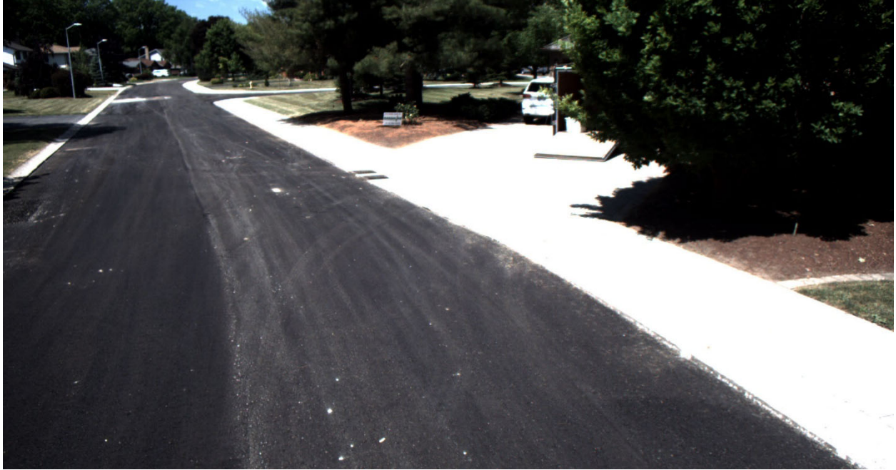
Pavement Condition Good – PCI 75 – 85
