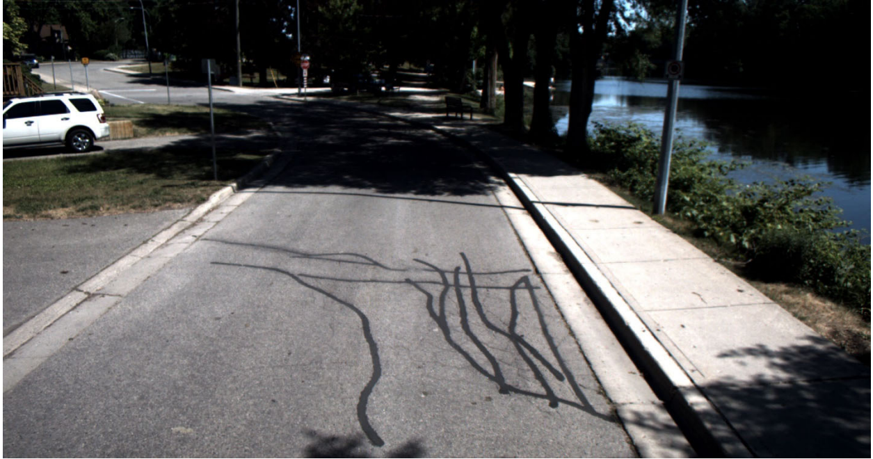
Pavement Condition Poor – PCI 40 – 57
