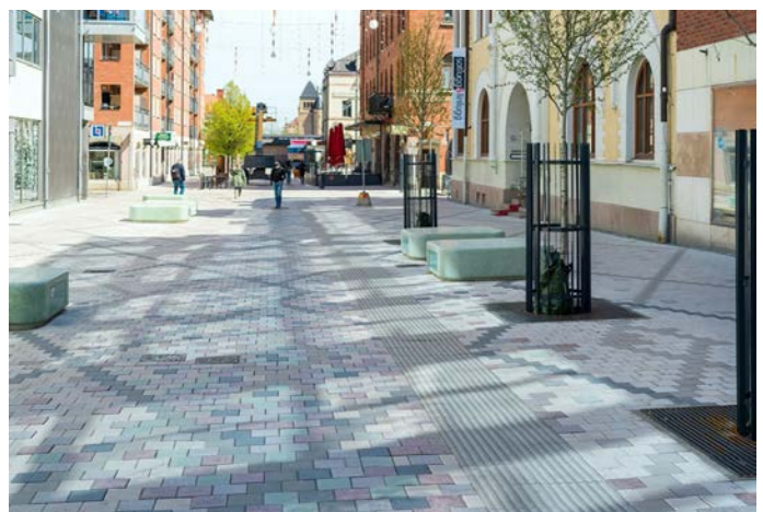
Precast concrete pavers and street furnishings in a public streetscape, creating a consistent identity.
