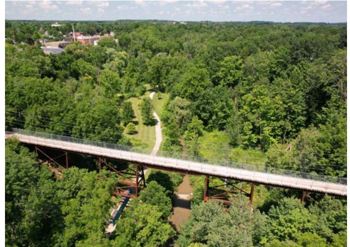
Aerial photo of Kinsmen Bridge
