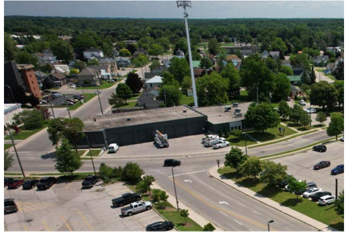
The existing Customer Service Centre, planned to be redeveloped into the new Town Hall location.
