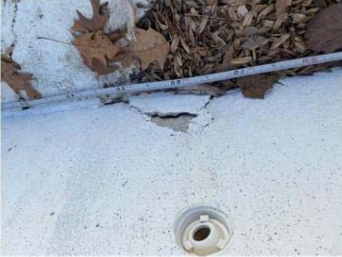
F. Special Construction - LLWP Pool Basin
