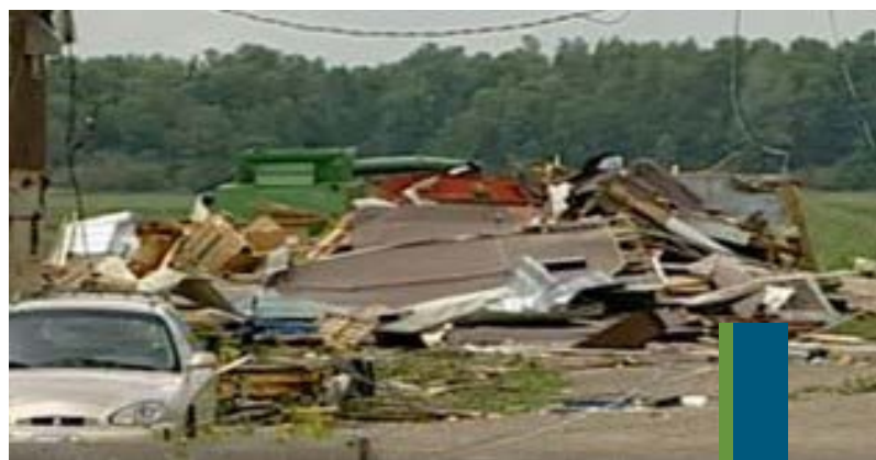
Figure 6: Damages from the August 2005 tornado in Southern Ontario (The Weather Network, 2021).
