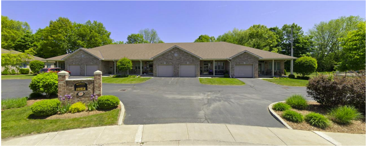
Figure 7 – Example of Townhouse Dwelling located at Balazs Court
