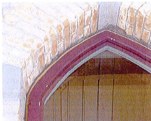
Figure 8, Brick arch with white penciling treatment.
