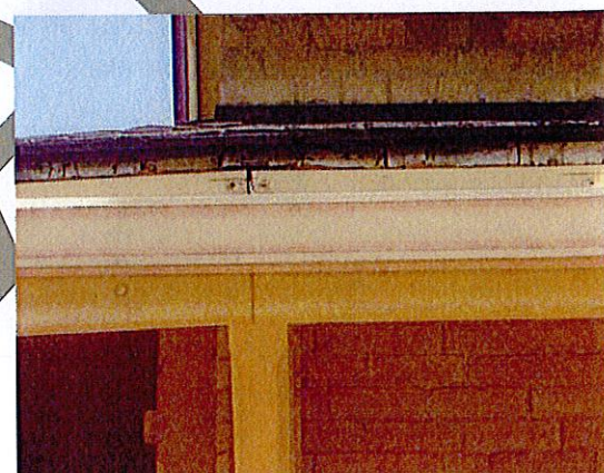
Figure 6, Exposed deck boards no drip flashings.
