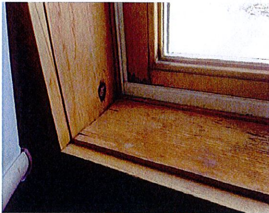
Figure 20, Water staining and sill deformation.
