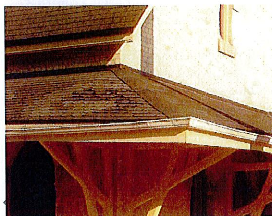
Figure 5, Sagging canopy roof and deteriorate shingles.
