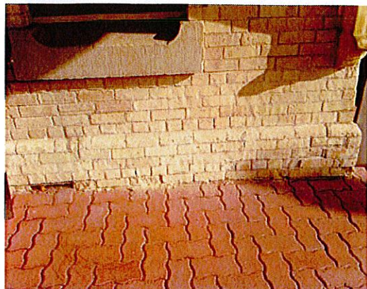
Figure 9, Deteriorated bricks at base of building.
