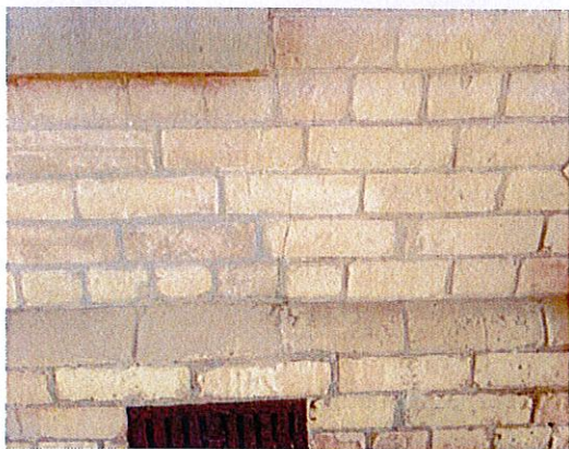
Figure 10, Diagonal cracking, inconsistent mortar repairs and brick mortar patch.
