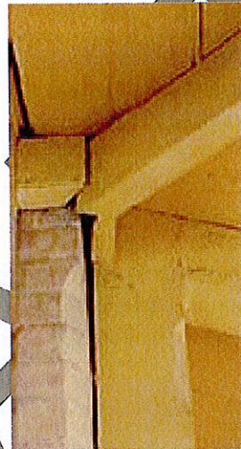
Figure 26, Separation at hip rafter connection.
