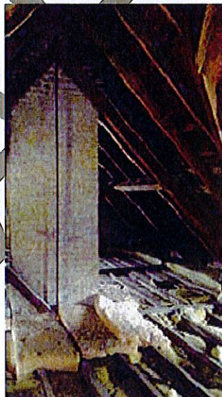
Figure 23, GWR station attic missing truss web.
