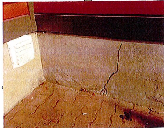
Figure 30, TLEPR station foundation crack.
